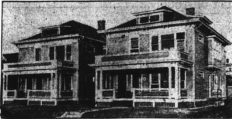
The trend of flat and apartment dwellers to the West End residence district of Tacoma is aptly illustrated in these new flats nearing completion for I. P. Wilson at 510-514 South O street. The houses are replica of each other and modernly equipped. Each is 28x33 feet in size, the subdivisions giving four five-room apartments. Large fireplaces finished in white Scotch brick, specially imported, add to the interior. Mr. Wilson has erected the buildings as an investment for himself and two daughters, Misses Kelly V. and Bertha L. Wilson. The cost was $6,000.
