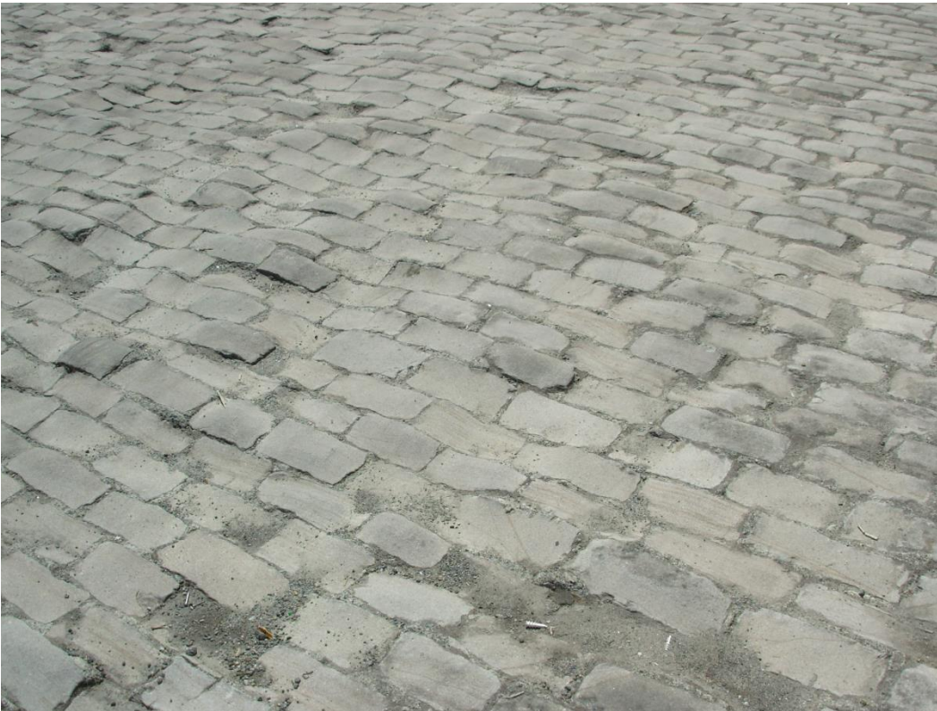
5 of 6 – N 11 th Street at 1000 Block, detail of sandstone pavers showing condition.
