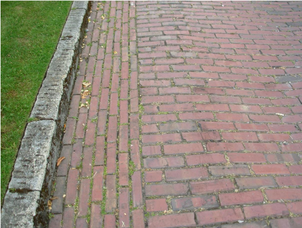
2 of 6 – N 9 th Street at 900 Block, Detail of brick gutter and curb.
