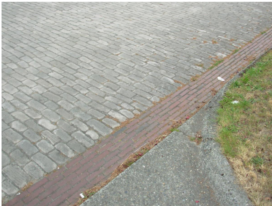
6 of 6 – N 10 th Street at 900 Block, detail of sandstone pavers and brick gutters.
