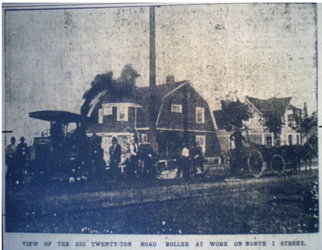
Bituminous macadam paving on North I. Picture at N. I and N. 9 th Streets. Tacoma Daily Ledger , 10/12/1902.
