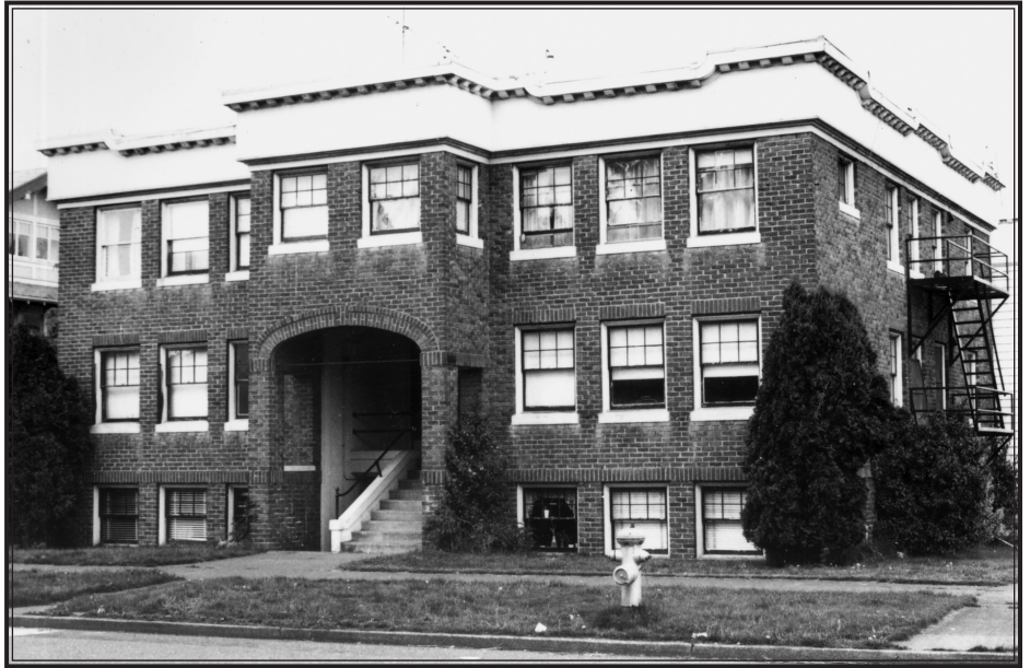
901 North M Street • Tacoma Public Library, BU-955
